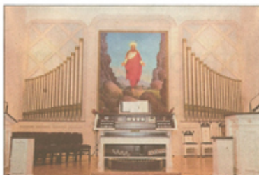
A renovation in Moravian Church, New Dorp, included building pipe organ chambers on either side of the rear wall for 24 ranks containing 2,000 individual pipes. PHOTO COURTESY OF JACOBSON CONTRACTING INC.
