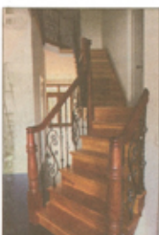
Wrought iron handrails are among the notable features of a renovation on Lighthouse Hill that required new construction. ADVANCE PHOTO/IAN SOMMER-HAMMILL
